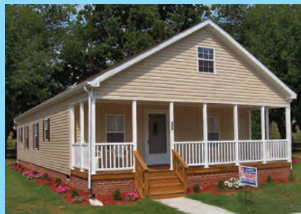
The finished product, a brand new, three-bedroom, two-bath, manufactured home.
