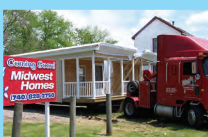
The 1,312 sq. ft. manufactured ranch home is delivered to its foundation at 929 Keen St. in Zanesville, OH.
