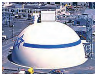
Lone Star Northwest Inc., in Portland, OR, uses a dome for dry powder cement storage.
