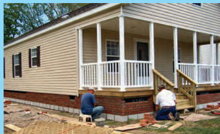
Workers complete the detailed brick work and other finishing touches on site.
