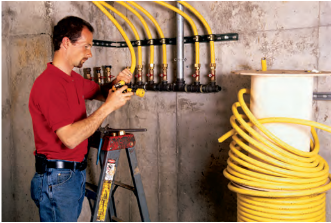
Builder Chris Meinhart makes flexible gas piping connections at the manifold at a custom home he was building in Willistown, PA. Each of the 3/4" Gastite lines coming off the manifold leads to a different gas fireplace or appliance.
