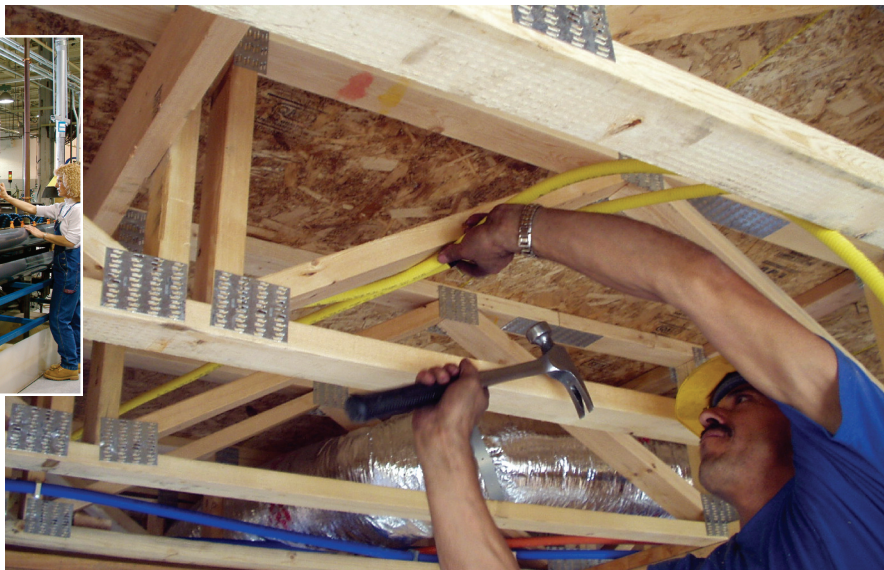
Great flexibility of Gastite's tubing enables swift installation around the multiple obstacles found in modern homes and commercial buildings.
