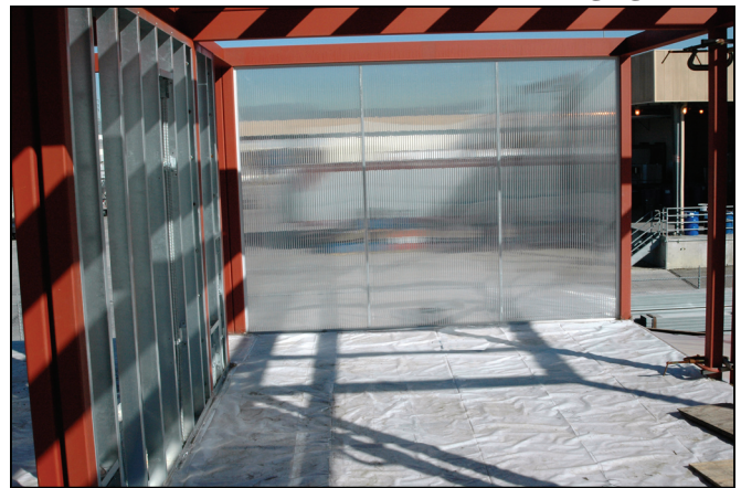
View from the second floor sun-room with pre-installed sub-framing and translucent Plexiglas wall. (Top)
