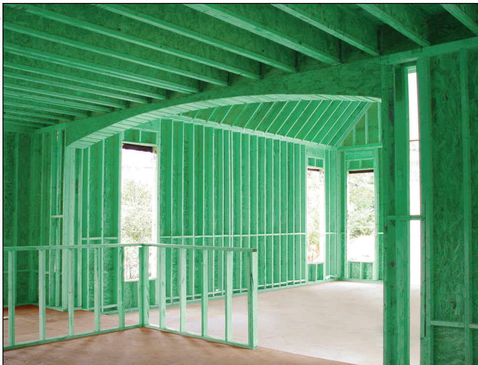
Distinctive green color indicates wood products are coated with FrameGuard protection against mold, mildew and termites.
