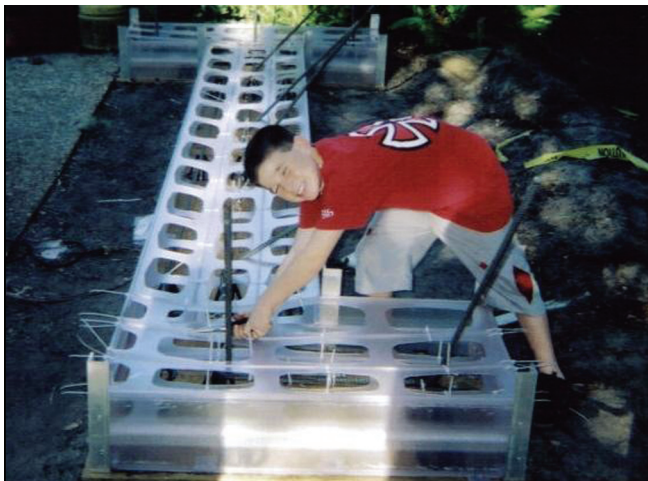
To drive home the point, regarding how easy the CPU system is to use, Lanc shows his grandson, Trevor, how to attach the center inserts and tie re-bar together with plastic-ties.
