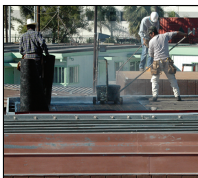
Workers hot-mop the roof of a reusable modular before releasing it to renters for a temporary site.
