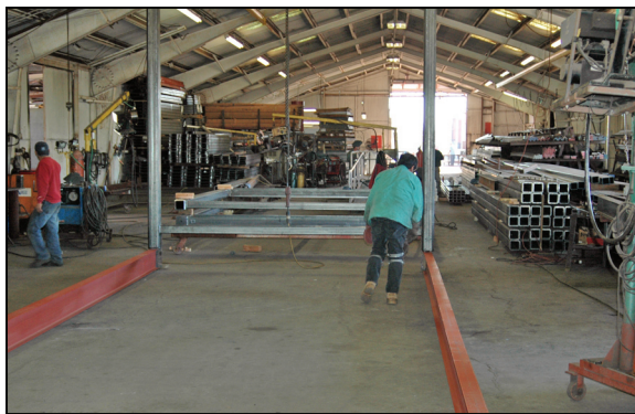
The first modular of a new custom design takes the longest, says Ortiz, the next 35 units will be a breeze.
