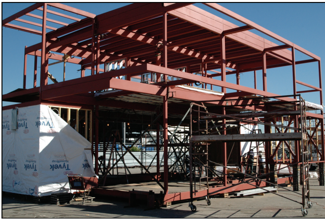
The entire custom structure is meticulously assembled at the plant and examined before being transported to its residential foundation site.
