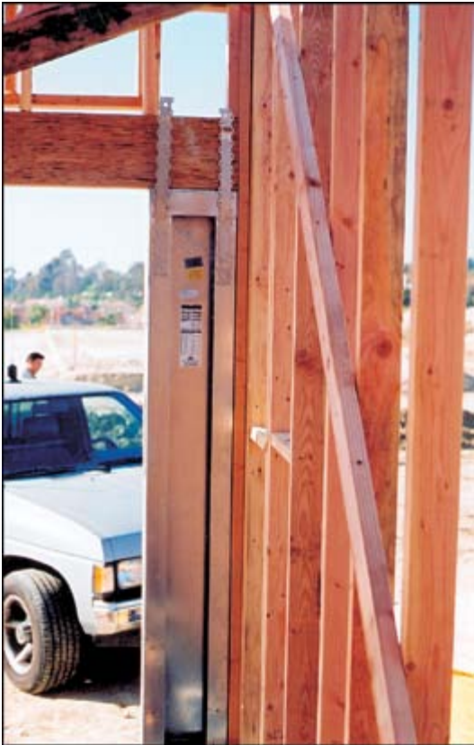
The HardyFrame panel can be easily integrated with wood framing and offers design flexibility and strength.
