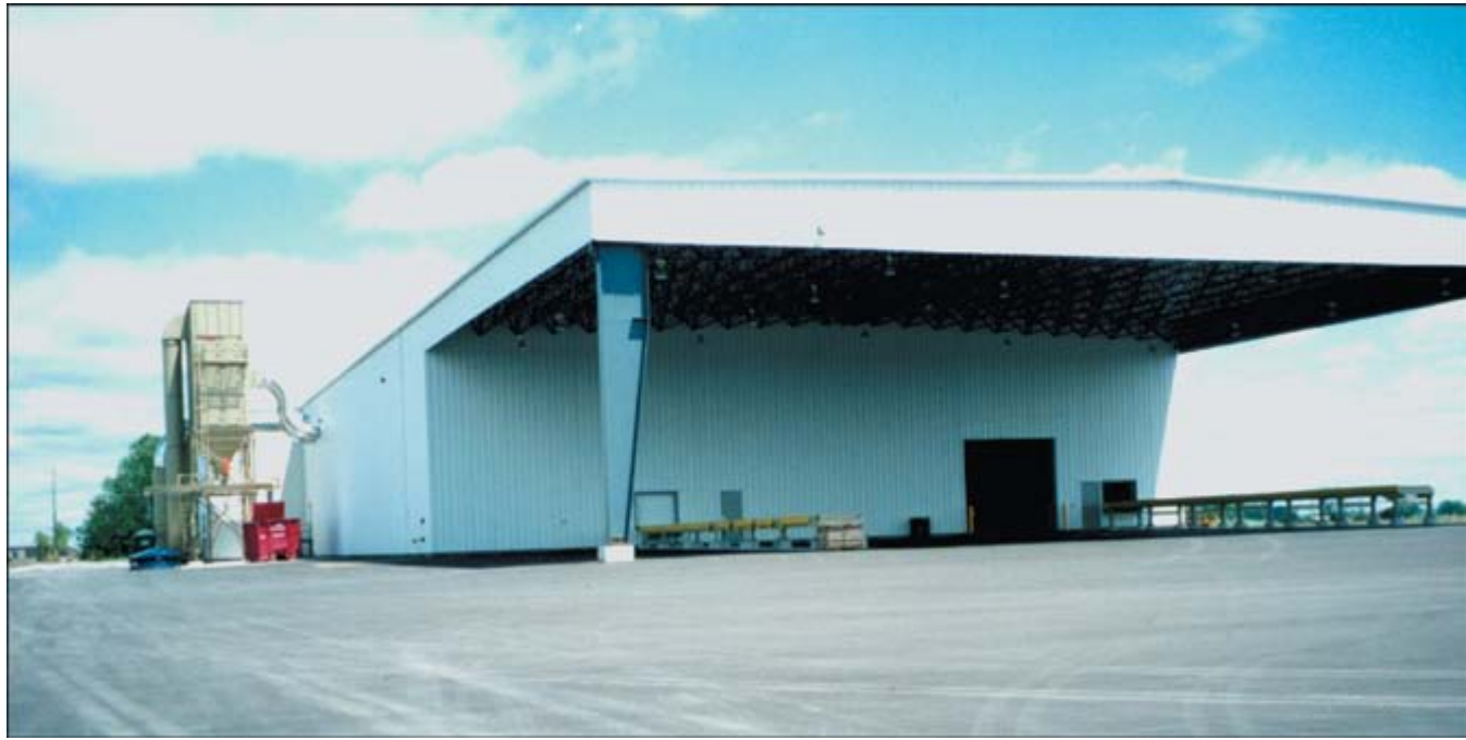
Jager completed construction of this wood I-beam facility in Bolton, ON capable of producing 50 million lineal feet per year .
